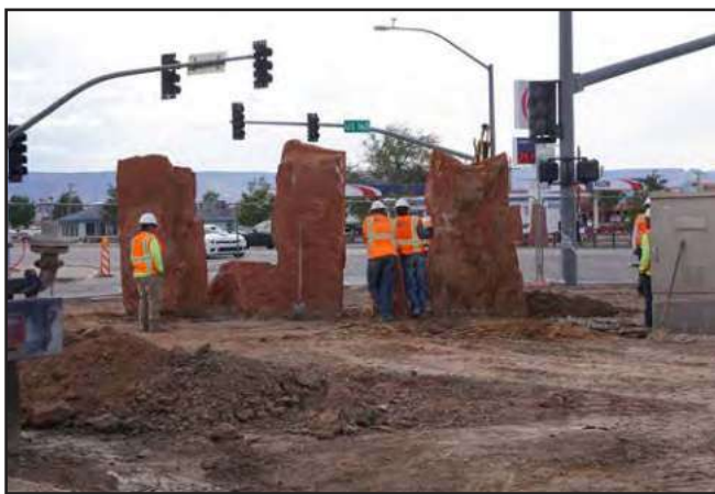
KAYENTA, ARIZ. MORNING DEW LANDSCAPING SET UP STONES
