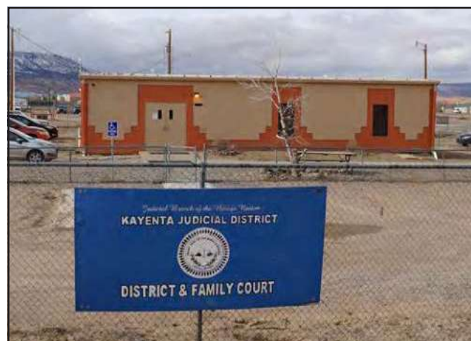
KAYENTA, ARIZ. THE CURRENT KAYENTA JUDICIAL COURT BUILDING
