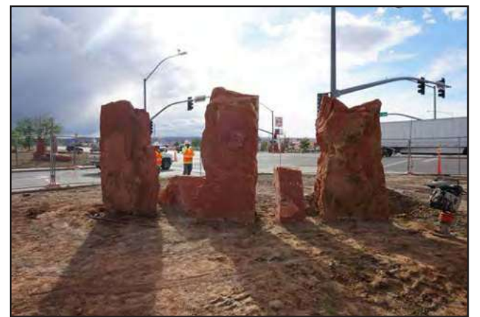
KAYENTA, ARIZ. ALMOST NEAR COMPLETION.
