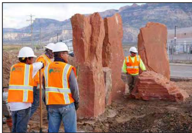
KAYENTA, ARIZ. LARGE STONES ARE PLACED IN STRATEGIC LOCATION.
