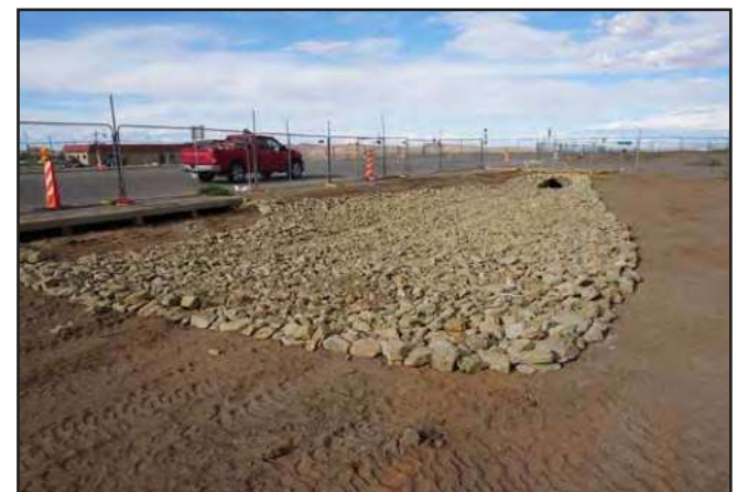
KAYENTA, ARIZ. CREW WORKING ON IRRIGATION FOR RUN-OFF.
