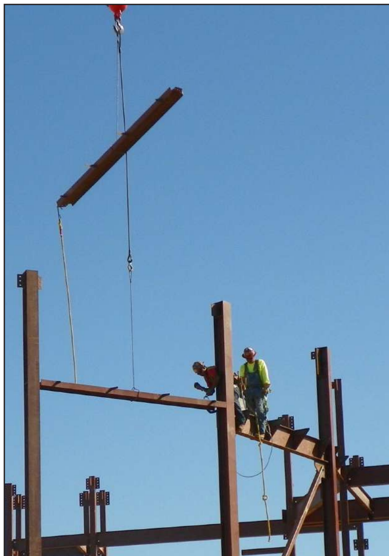
Iron workers installing iron beams high above the ground at the new Kayenta IHS Hospital Site. Photos & Blueprints: Flintco, INC.
