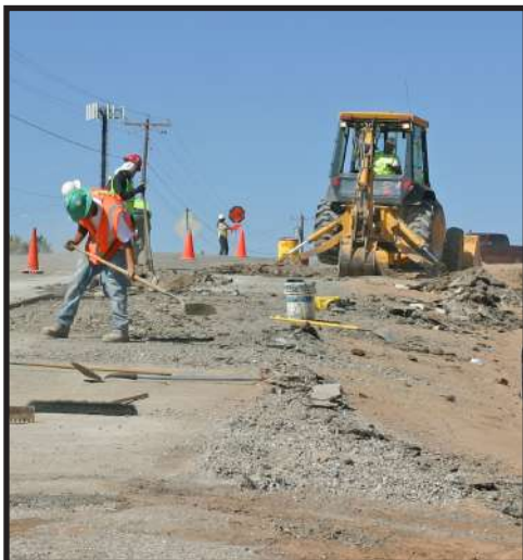
Township workers repairing the road to Wetherill Heights.
