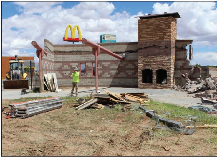
KAYENTA, ARIZ. - Workers taking down CMU walls of the structure.
