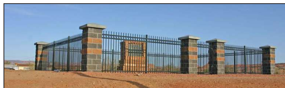
Wetherill site after renovations.
