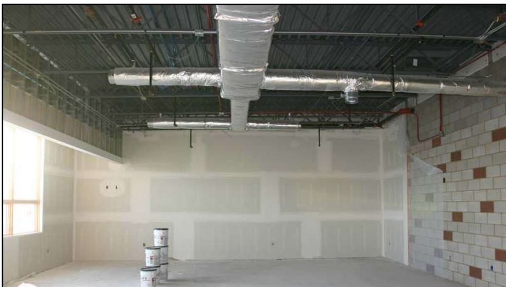
A new large classroom is ready and waits for paint and texture.
