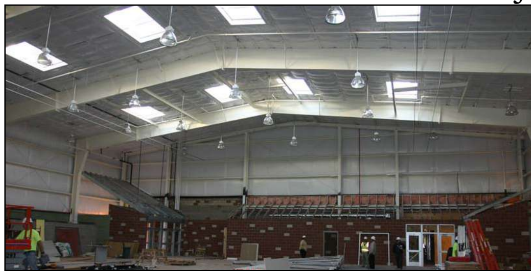
The new KCS gym nears completion. Skylights drastically improve lighting in the complex.
