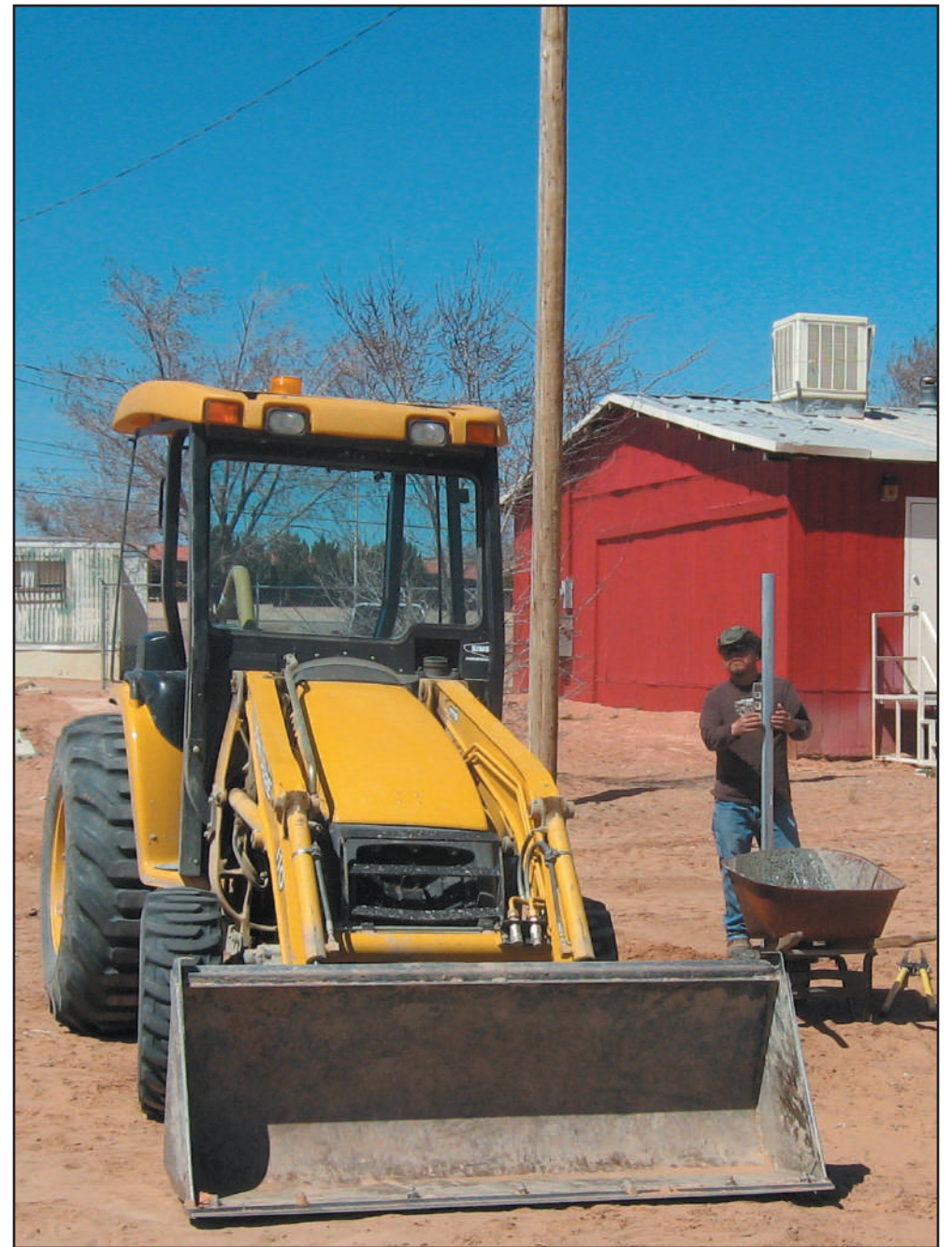
Kayenta Township Construction Crew working Senior Center Fencing project.
