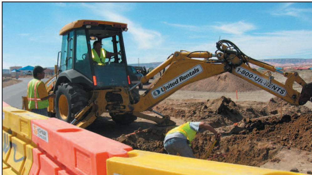
Keyah Construction working on sewer line project.
