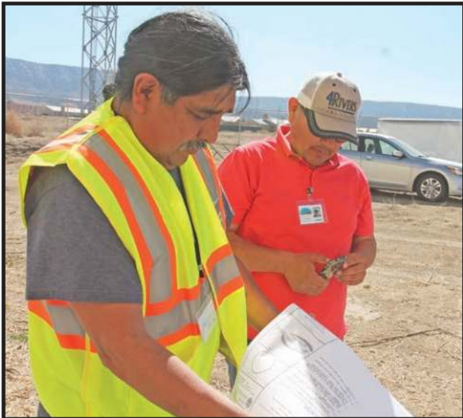
Kayenta, Ariz. - Community Development and Public Works identifying sewer line location at Kayenta Police Department. (Photo Chris Burnside, KTC.)
