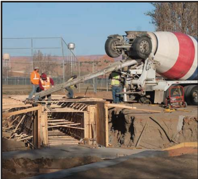
Kayenta, Ariz. - Community Development providing field inspection at KUSD cattle guard. (Photo Chris Burnside, KTC.)
