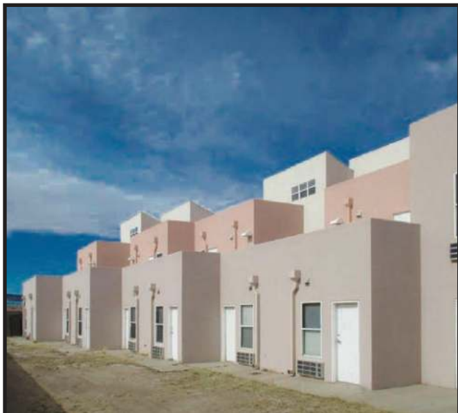
Kayenta, Ariz. - Kayenta Township Community Development and Public Works assisting with inspections at Tohdenasshai Shelter Home. (Photo Courtesy of Mark Joseph, KTC.)
