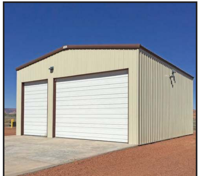
Kayenta, Ariz. - A complete 'Snow Removal Equipment' Building fully functional with power and landscape. (Photo Chris Burnside, KTC)
