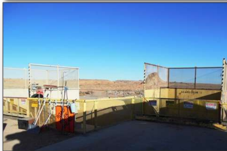
The Kayenta Township's transfer station is the only one within the Kayenta-area and it operates with one dump truck, two compactors, four stationary dumpsters and an oil recycling tank.
