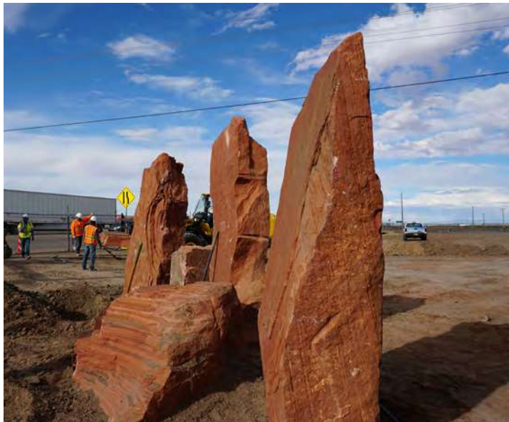
KAYENTA, ARIZ. BEAUTIFICATION PROJECT AT US HWY 160 & 163
