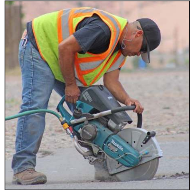
Kayenta, Ariz. During the Summer, Public Works Department have been working on maintaining some of the streets. Shown is Bradley Boaz Blair cutting asphalt for repairs.
