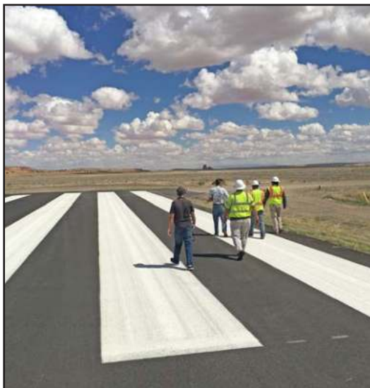
Kayenta, Ariz. A crew inspect the airport landing strip. A walk through with KTC Building Inspector and Project Coordinator assist with inspection of final walk through, making sure work is done properly.
