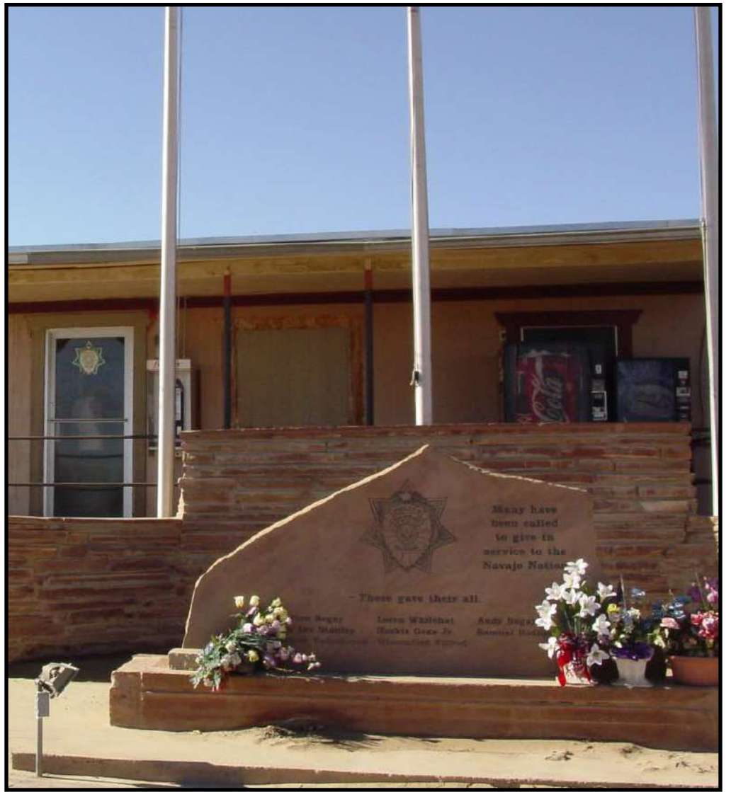
Kayenta's current Police Department will be replaced by a 7,155 square foot building.
