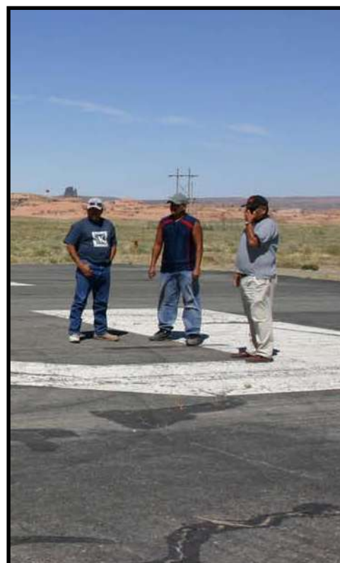
Bill Cly and Kayenta Township Maintenance survey an area of the runway for repair.
