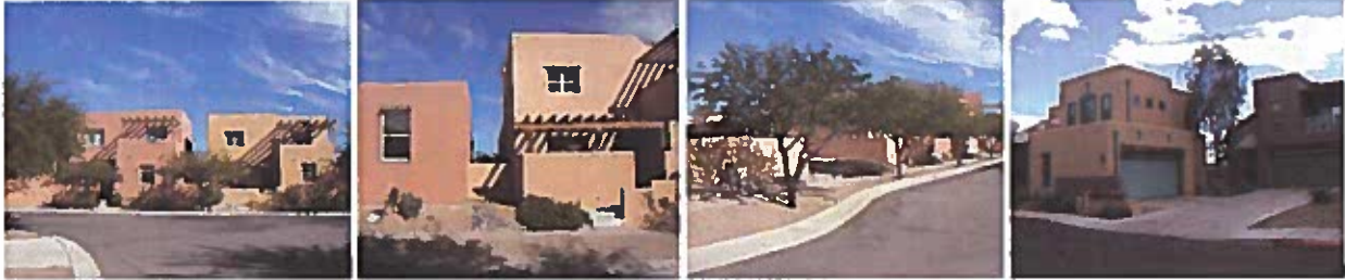
Variety of Single Family Energy Efficient Homes in Close Proximity to Transit, Employment and Civic Center
